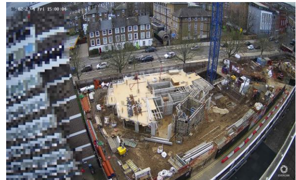
Block B Progress – Herdwick House
