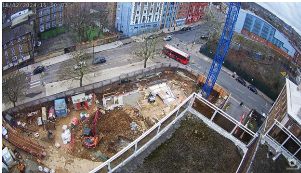
Block A Progress – Swaledale House
