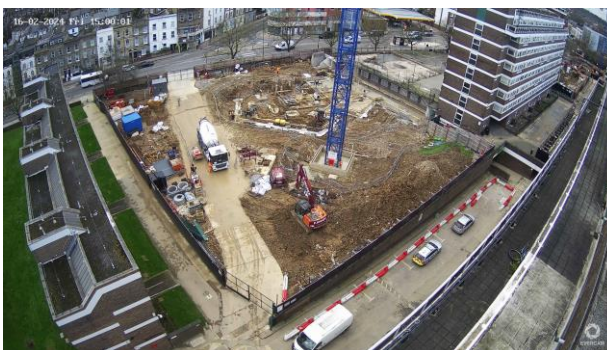
Block C Progress – Ryeland House
