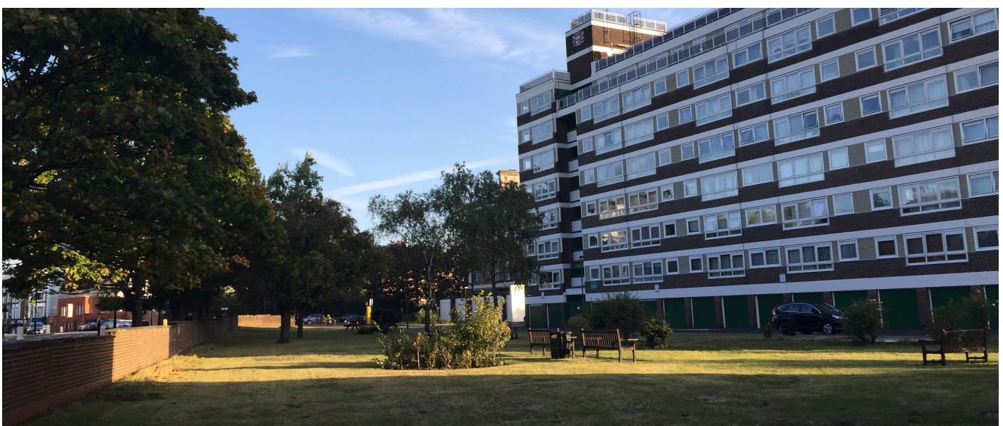
Space C - Lambfold House Green, York Way Estate
