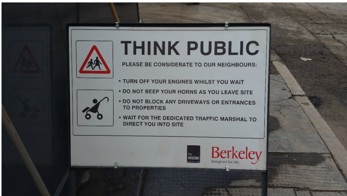
Figure 2: Simple measures such as signage at the site entrance can inform driver behaviour
